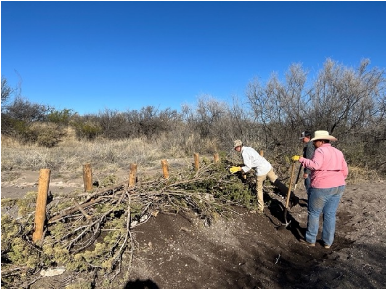
Figure 51. Sul Ross State University Students visit the Alamito Creek Preserve during a field trip for their Hydrology course to help install experimental brush weir structures with the Rio Grande Joint Venture. (Photo by Philip Boyd)
