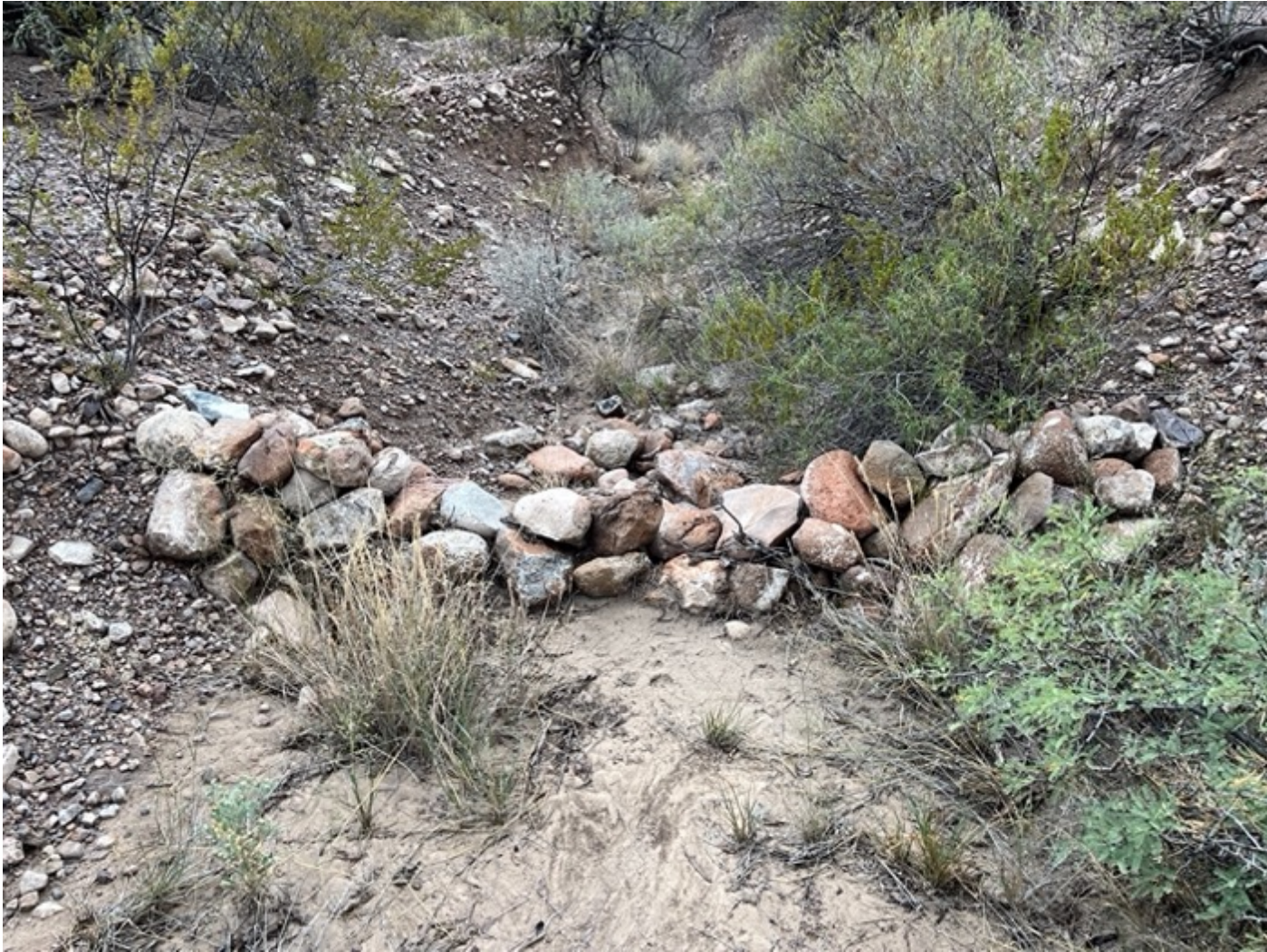
Figure 49. Photograph taken November 2023 facing downstream from the upstream side of leaky rock structure built in 2021 on the Alamito Creek Preserve. This photo shows newly piled sediment on the upstream side with grasses growing through the soil. These structures are examples of low-tech approaches to restoring eroded sites as they help slow water and capture sediment that would normally be carried away in runoff.
