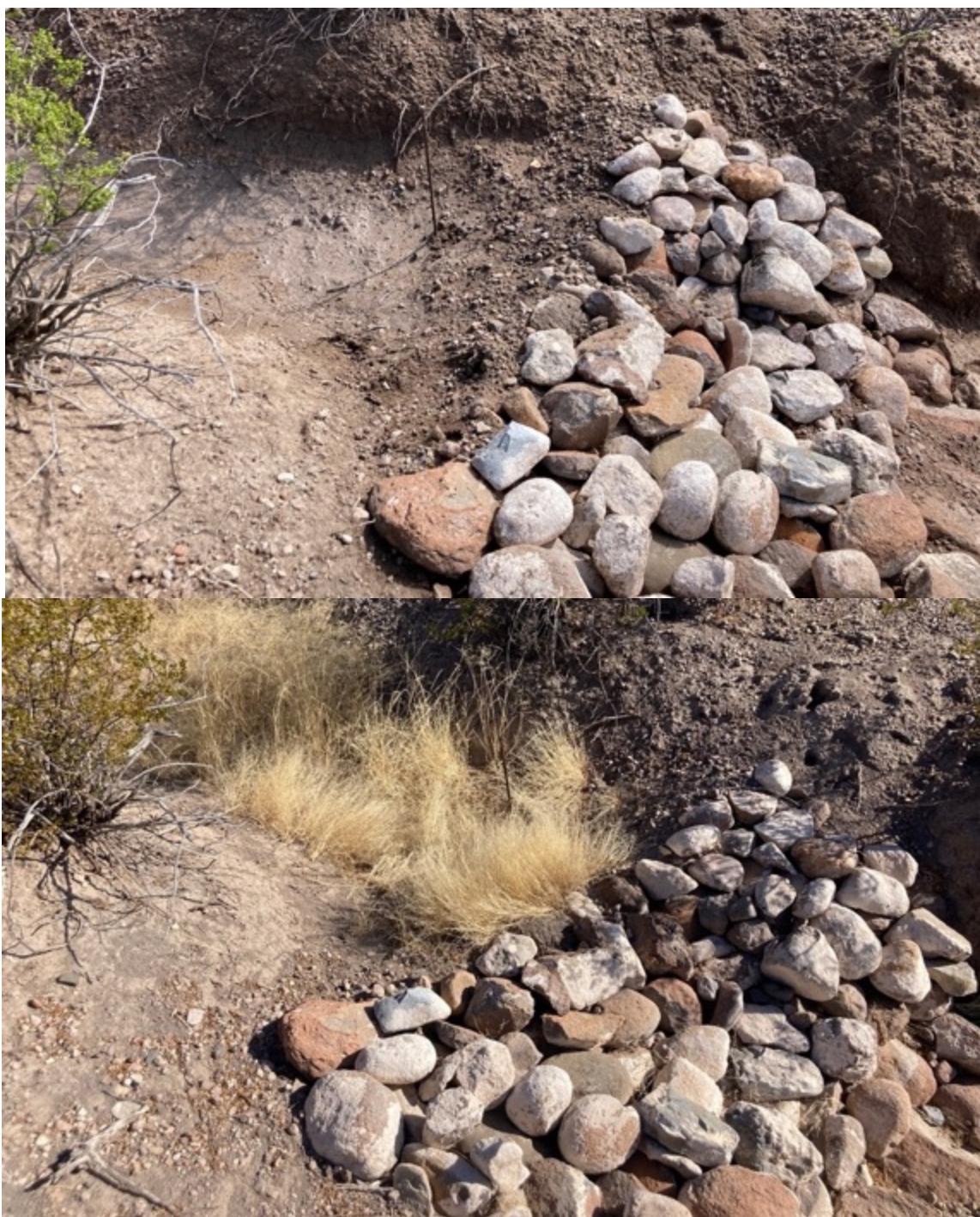
Figure 48. Photographs of a leaky rock structure built in April 2021 on the Alamito Creek Preserve.. The top photo shows the structure one month after construction and after a recent rain. In 2023, new plant growth on the upstream side of the structure can be seen (bottom photo) where water has been slowed and sediment has been dropped and collected. (These structures of examples of low-tech approaches to restoring eroded sites as they help slow water and capture sediment that would normally be carried away in runoff).
