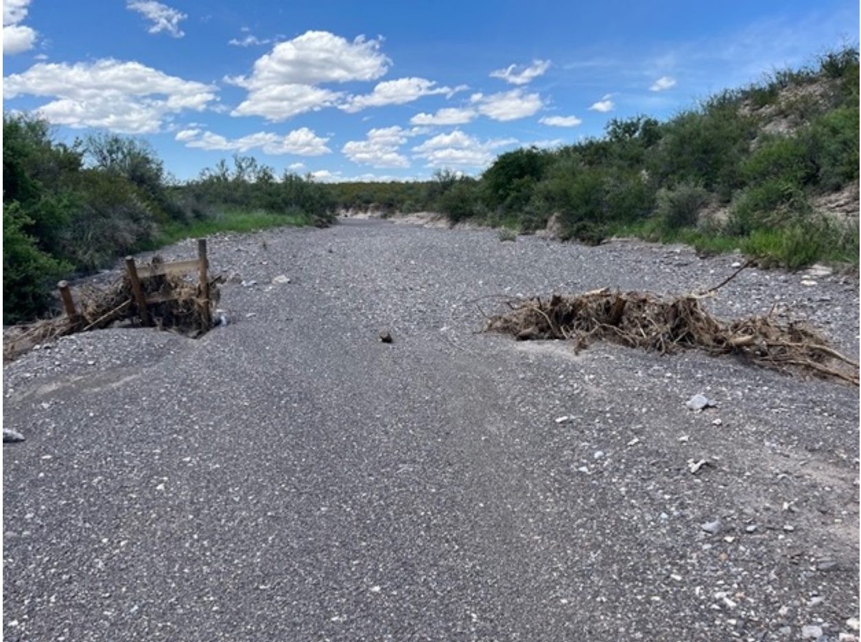
Figure 53. Photograph showing the aftermath of a late-May 2023 flood in Matonosos Creek on the Alamito Creek Preserve. Several brush weir structures were built by the Rio Grande Joint Venture and Dixon Water Foundation with the intention of slowing water down to improve hydrological function, reduce runoff, and improve riparian habitat. This flood proved to overwhelm the structures as they were installed. The organizations plan to evaluate lessons-learned and attempt a second round of structures in 2024. (Photo by Philip Boyd)
