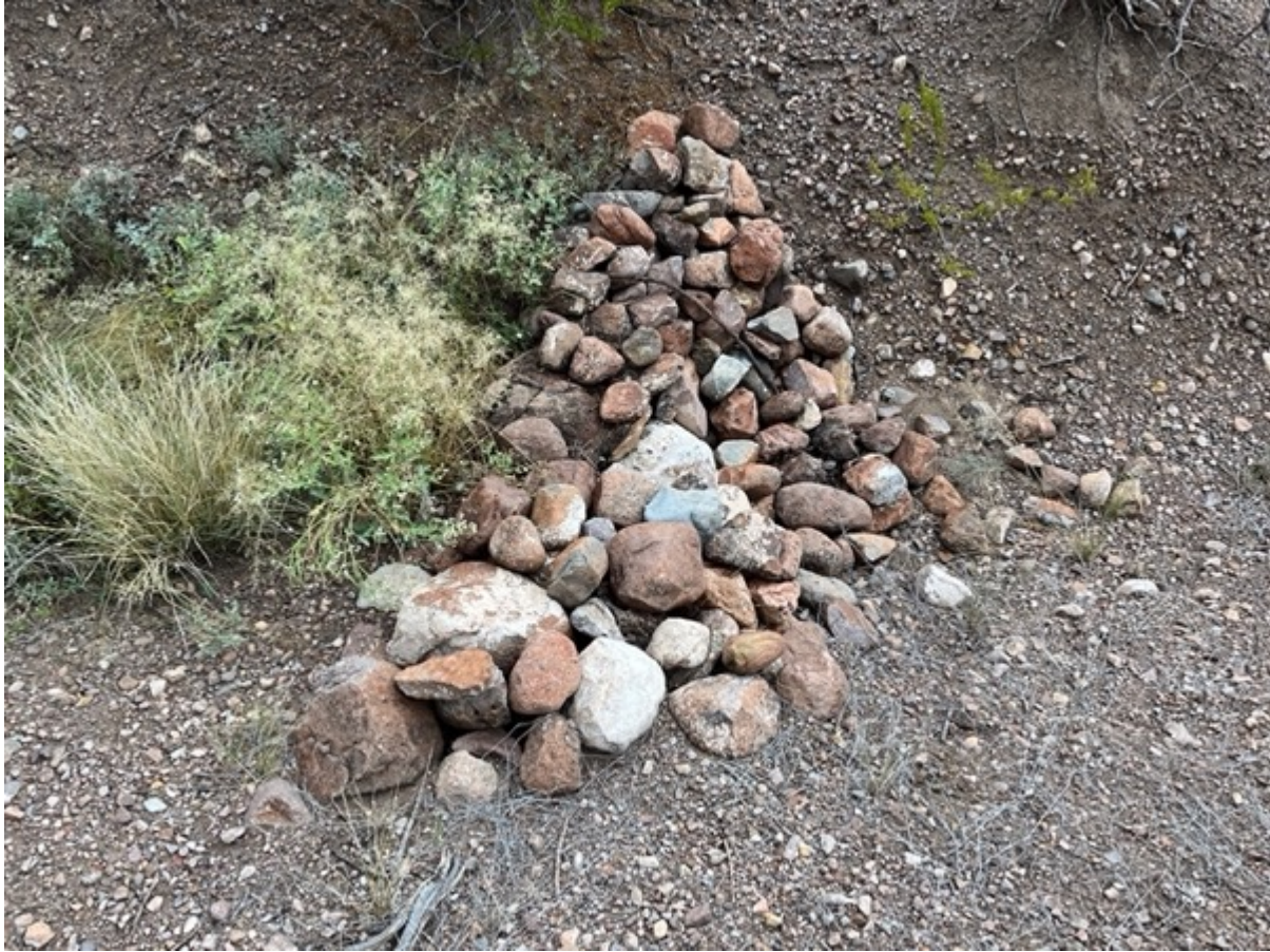
Figure 50. Grass grows behind a leaky-rock dam that was built in an incised tributary at Alamito Creek Preserve, April 2021. These structures allow water to filter through while also slowing the water, dropping sediment on the upstream side of the structure. This sediment also retains moisture for longer periods of time than a channel in which water passes through quickly during a flashing event. This photo shows the lifted channel in 2023, resulting from this sediment capture and the resulting vegetation that grew from these conditions in what was formerly an incised and bare channel. (Photo by Philip Boyd)
