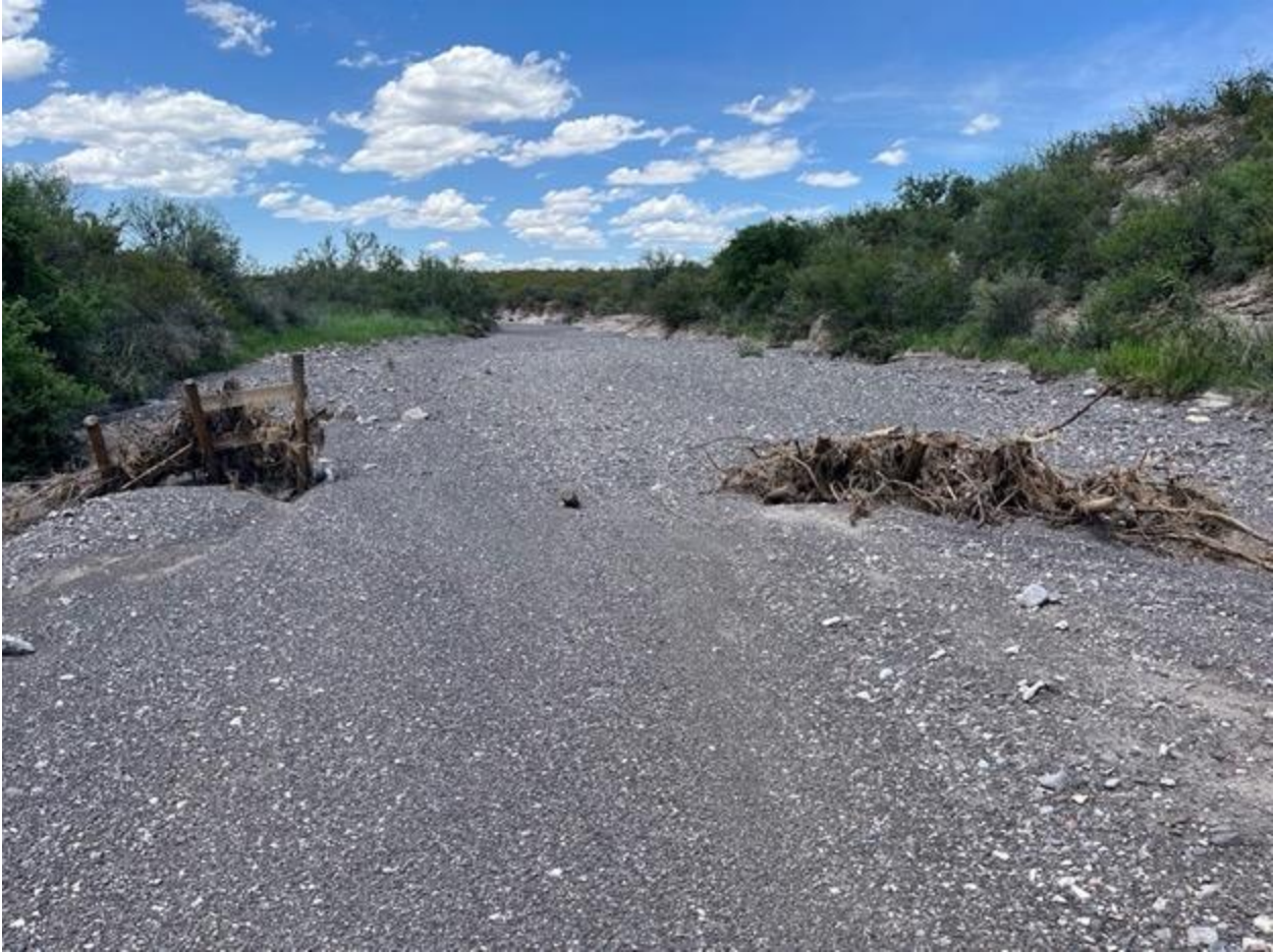
Figure 53. Photograph showing the aftermath of a late-May 2023 flood in Matonoso Creek on the Alamito Creek Preserve. Several brush weir structures were built by the Rio Grande Joint Venture and Dixon Water Foundation with the intention of slowing water down to improve hydrological function, reduce runoff, and improve riparian habitat. This flood proved to overwhelm the structures as they were installed. The organizations plan to evaluate lessons-learned and attempt a second round of structures in 2024. (Photo by Philip Boyd)
