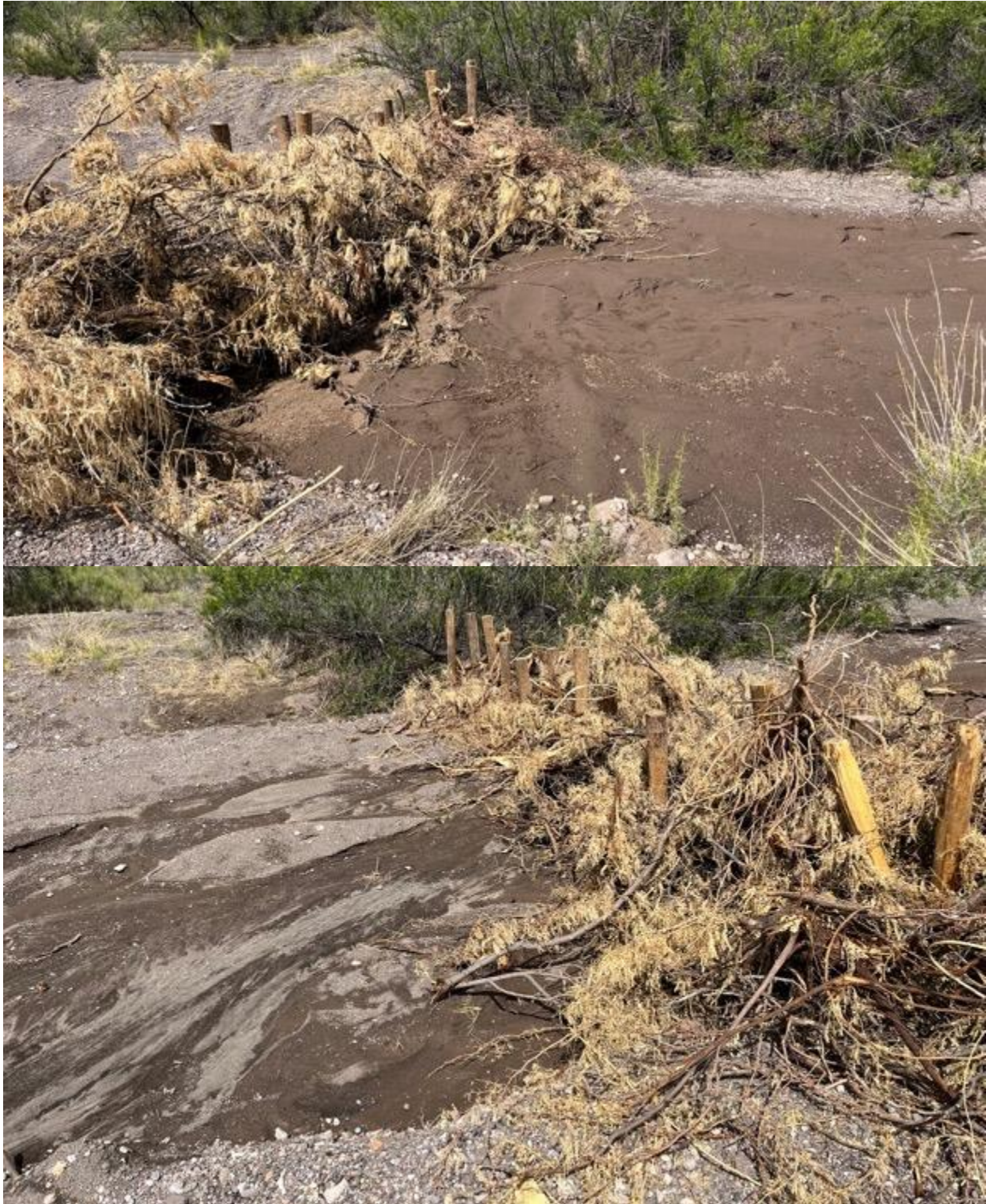
Figure 52. Brush weirs structures show uniformly-moist soil evidence of pooling, on the upstream side of structure (top) and more unevenly-moist soil on downstream side (bottom) after water has filtered through the structure after a mid-May 2023 flow event in creek. (Photo by Philip Boyd)
