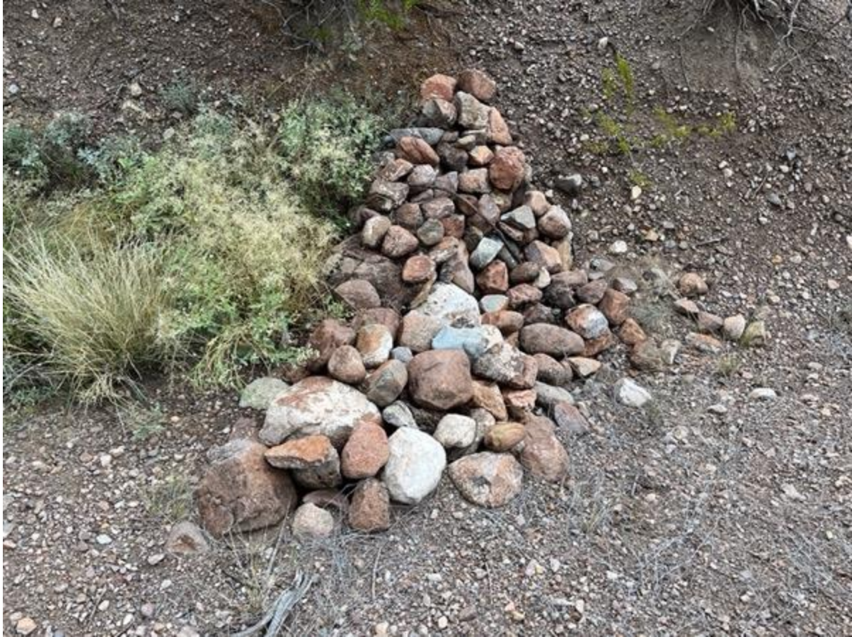
Figure 50. Grass grows behind a leaky-rock dam that was built in an incised tributary at Alamito Creek Preserve, April 2021. These structures allow water to filter through while also slowing the water, dropping sediment on the upstream side of the structure. This sediment also retains moisture for longer periods of time than a channel in which water passes through quickly during a flashing event. This photo shows the lifted channel in 2023, resulting from this sediment capture and the resulting vegetation that grew from these conditions in what was formerly an incised and bare channel. (Photo by Philip Boyd)
