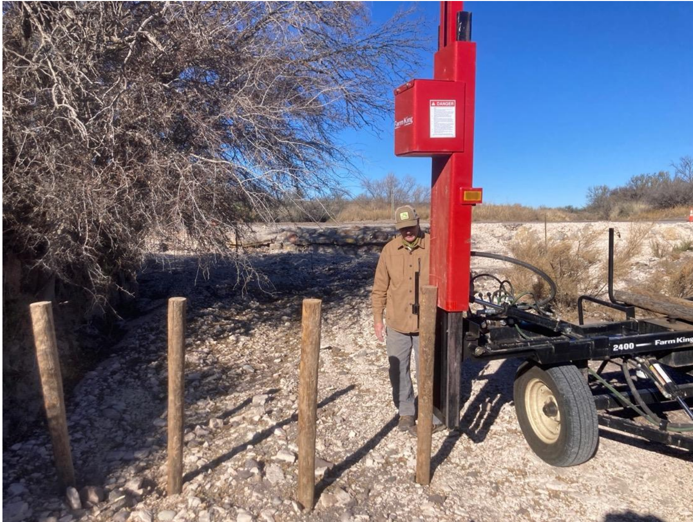
Figure 46. Rio Grande Joint Venture hydrologist Jeff Bennett using a hydraulic post pounder to install brush weirs in Matonoso Creek on Alamito Creek Preserve, October 2022. (Photo by Philip Boyd)
