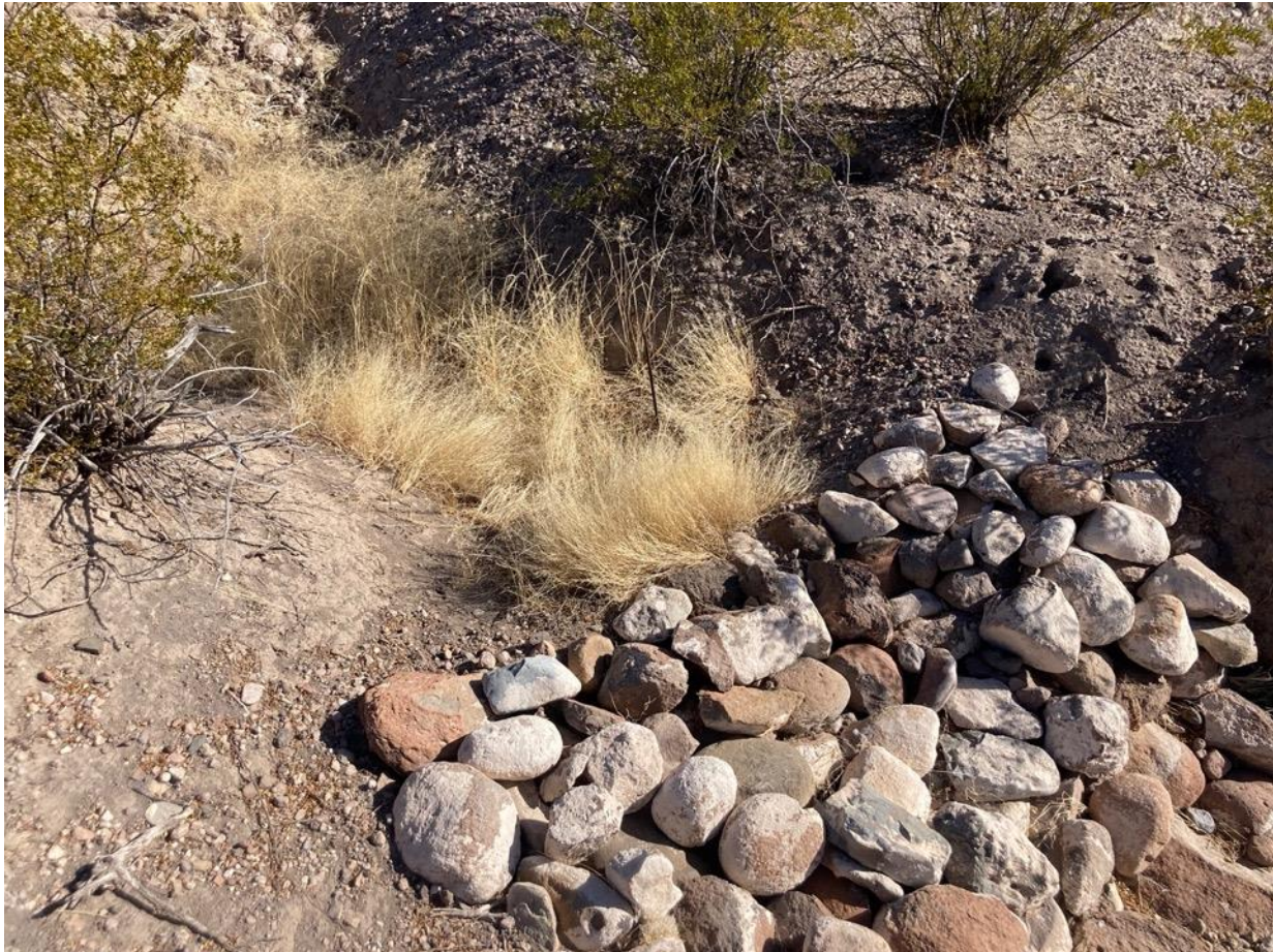
Figure 44. Grass grows behind a leaky-rock dam that was built in an incised tributary at Alamtio Creek Preserve, April 2022. The structure of loose rocks was built in April 2021 and allows water to filter through while also slowing the water, dropping sediment on the upstream side of the structure. This sediment also retains moisture for longer periods of time than a channel in which water passes through quickly during a flashing event. This photo shows the lifted channel resulting from this sediment capture and the resulting vegetation that grew from these conditions in what was formerly an incised and bare channel. (Photo by Philip Boyd)
