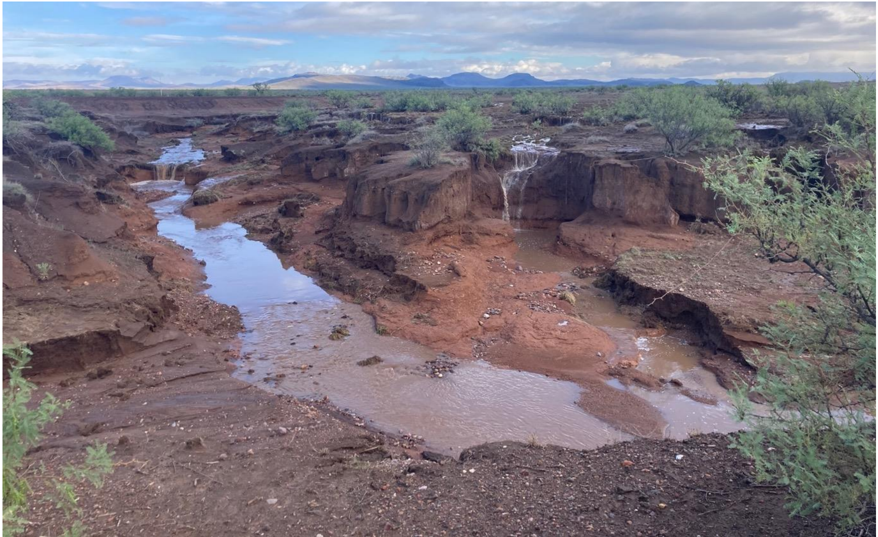
Figure 25. Just upstream from George erosion monitoring site, this photo shows water spilling around and over earth dam at knickpoints as floodwater works its way to the Alamito Creek bed below..
