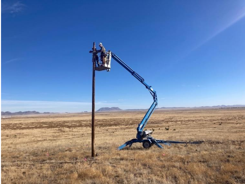
Figure 31. Bird Conservancy of the Rockies technicians prepping an out-of-service utility pole to be repurposed as a Motus tracking station on the Mimms Unit, December, 2021 (photo credit – Philip Boyd)
