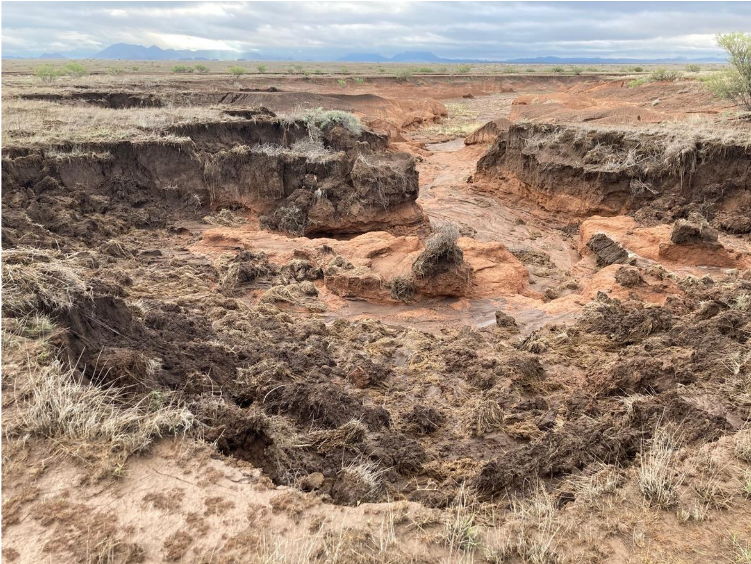
Figure 24. Erosion monitoring site showing evidence of bank collapse and soil loss soon after June 2021 floods (photo credit – Philip Boyd)
