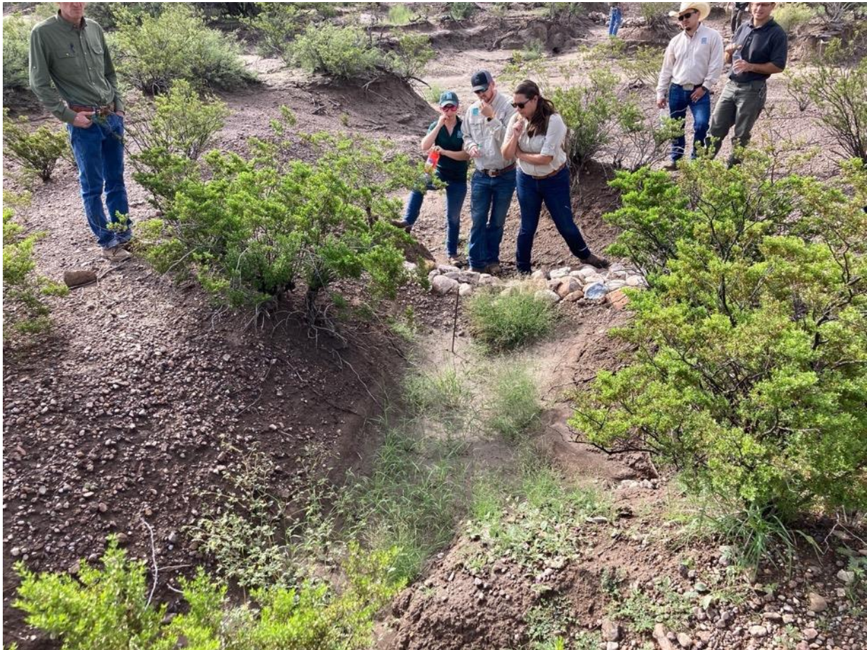
Figure 33. Texas Parks and Wildlife Department biologists and local land managers stand downstream from a leaky rock dam, installed in an eroded tributary channel April 2021, and view vegetation growing in caught sediment on the upstream side of the structure between April and August 2021.
